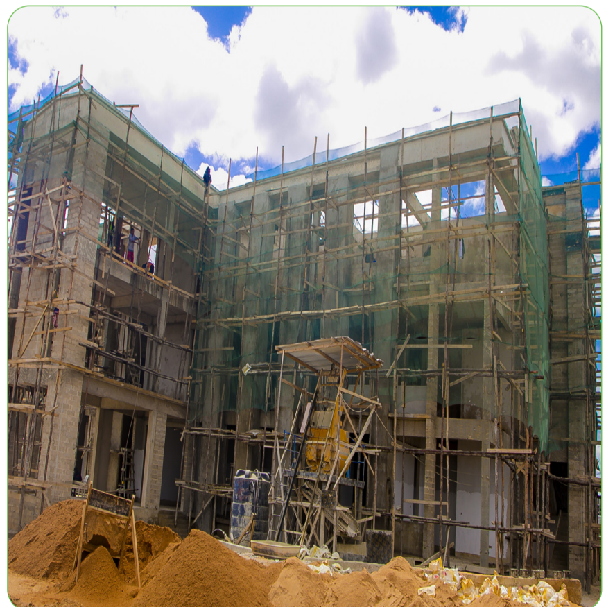
PPRA Head Office building under construction in Dodoma as on May 9, 2023
